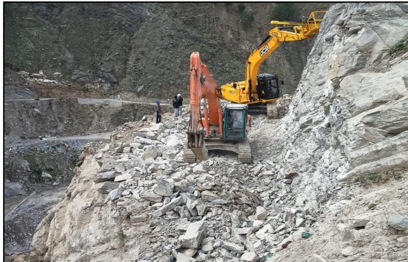
Dam Abutment Stripping
