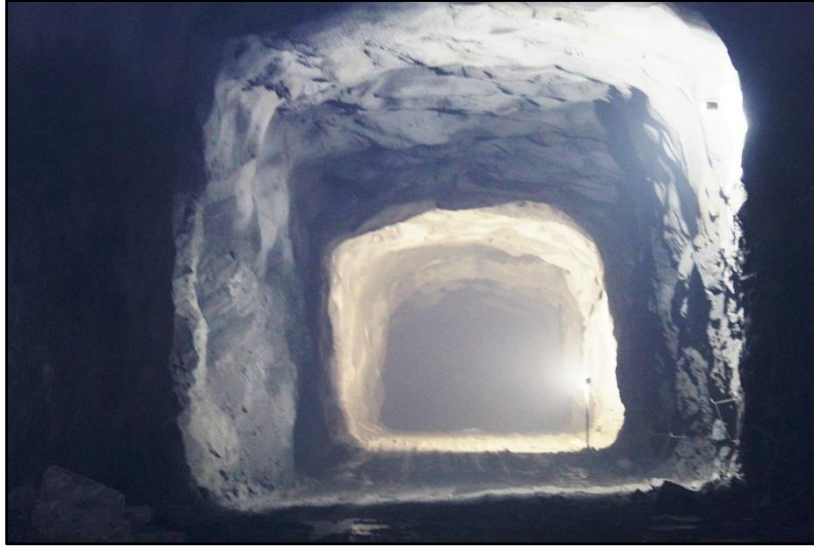
Power House Cavern Excavation
