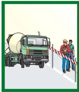
7. Precautions against vehicular traffic taken by barricading the area.
